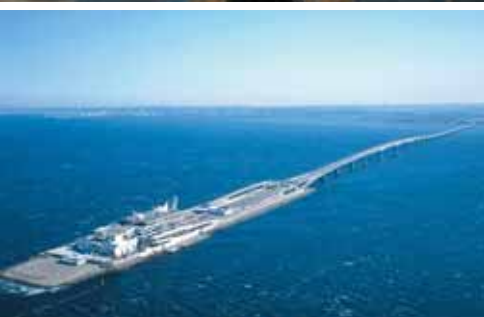
"Umihotaru", a parking area in the sea Tokyo Bay Aqua-Line Road
